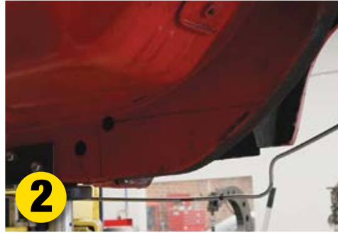
2 Measure, mark, check and confirm where you will cut the frame rails for your new front spring buckets.
