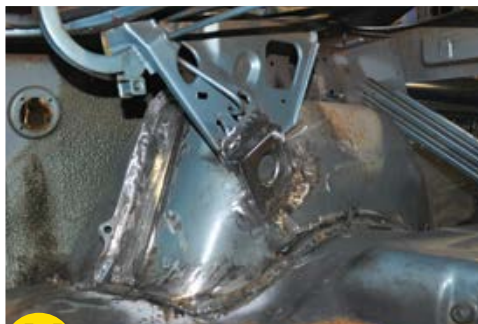
11 Be sure to weld the package tray brackets to your new widened wheel tubs and use the trunk hinge brackets in the kit to weld your trunk hinge brackets into place.
